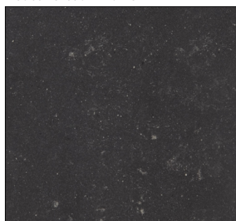
Internal Tile Floor
